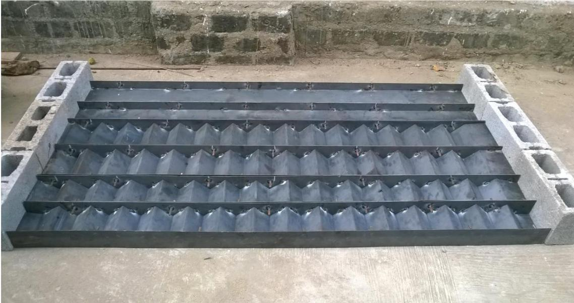
**Figure 2. Beams Placed For Casting**
